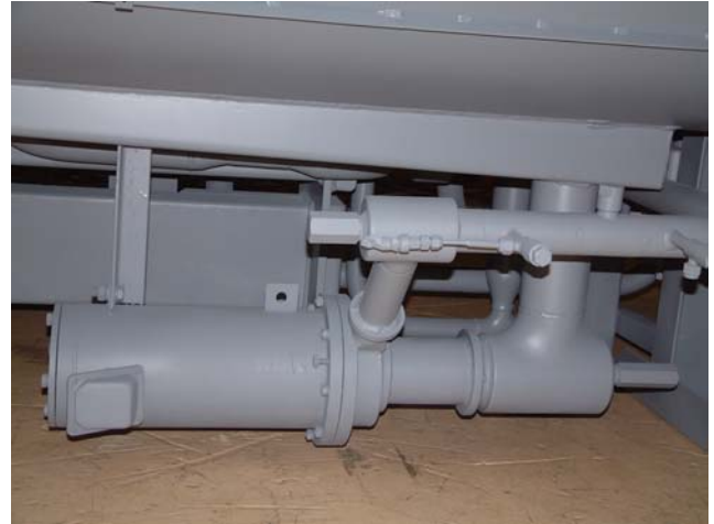
VIEW OF TYPICAL HERMETIC PUMP/MOTOR ASSEMBLIES
